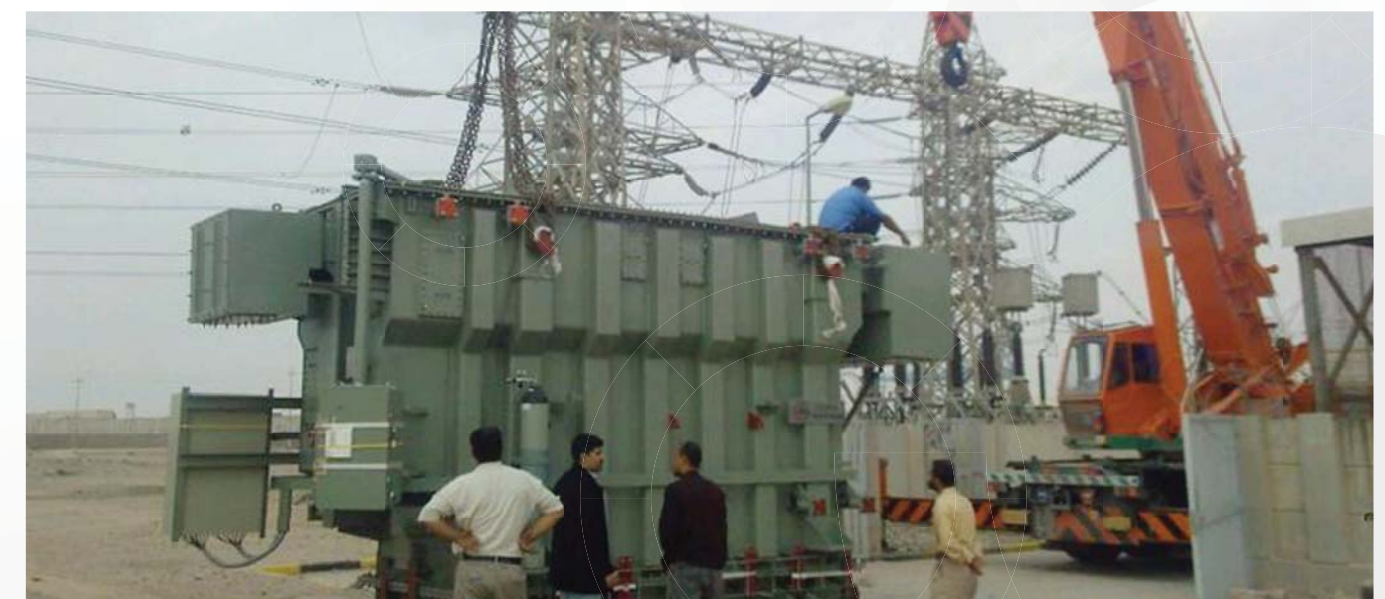
Transformer being erected at site (Iraq)
