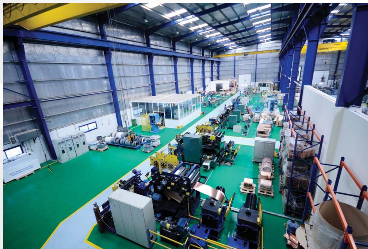
Inside view of the plant (winding section)
