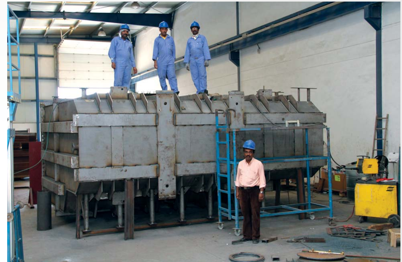
Power transformer tank
