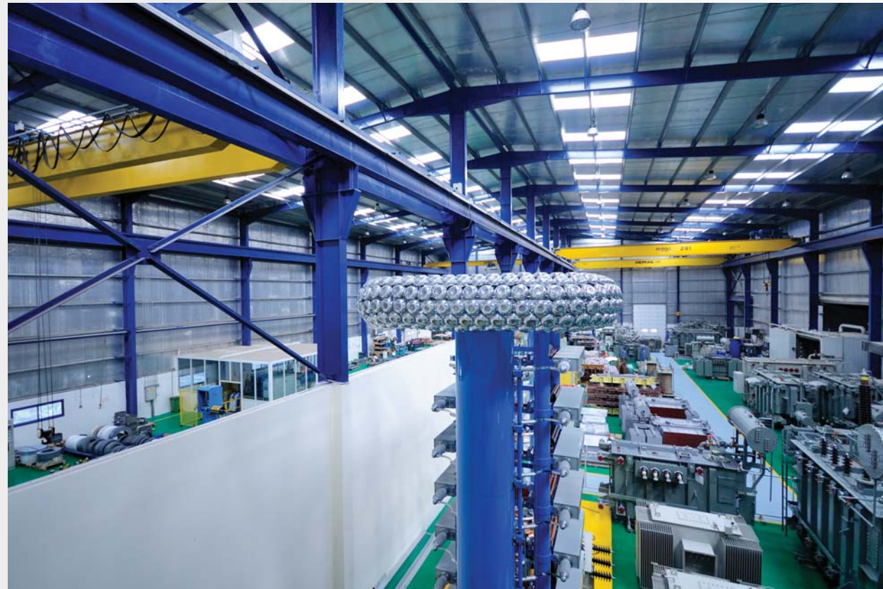
Inside view of the plant (test area)
